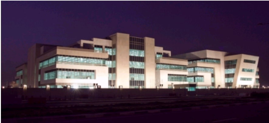
Ooredoo's next generation Smart Data Center 'QDC5' at Mesaimmer, Qatar (Photo: Business Wire)
