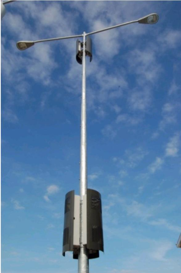
The new CommScope Metro Cell Concealment Solution features a two-piece design for mounting all the necessary equipment for metro cell operation, making for a total solution. Two aesthetically pleasing enclosures can mount and hide radios, antennas, backhaul termination (wireline or wireless), back-up batteries and other equipment on street poles in units that are more structurally balanced and easier to permit.
